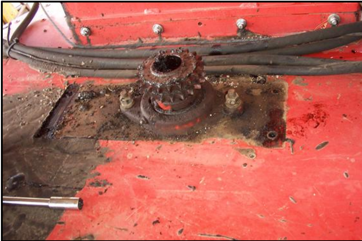
Fig. 6-5 Removal of Motor Mount Assembly
